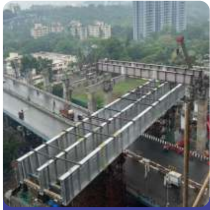
Assembly & Erection Of Girder
